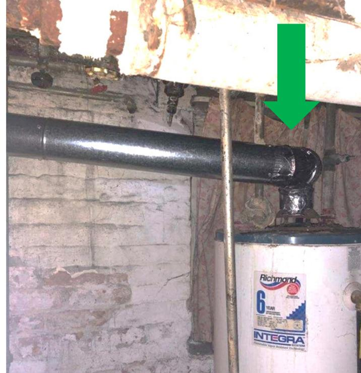
Disconnected flue vent for the water heater. Deadly carbon monoxide is being emitted to the basement when it should be vented to the outside.
